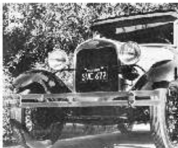
Bumper with flat rounded, open end, without the usual bolt, is one of the more obvious features of a true "early bird." Also notice round center bumper clamp with Ford script and "made in USA" - same as Model T
