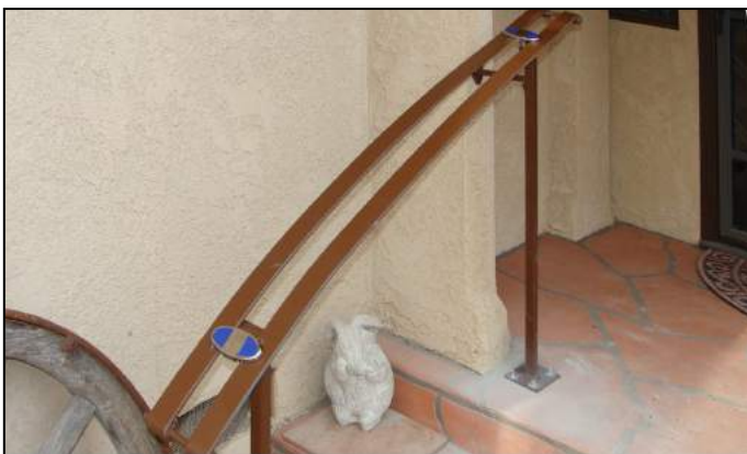
This may not be a car photo but may still have interest. I made a hand rail for the entrance to our home.....for our Model A friends. I got the idea...my wife modified it and together we worked out details to make it work. I started with a single bumper but could not make it come out ok. She came up with the solution. Bill and Jan Ewertz, Sonoma CA
